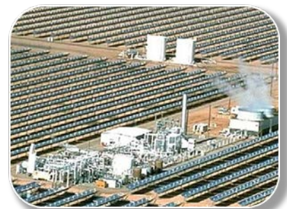
Kramer junction – view of the power block from the SEGS project
